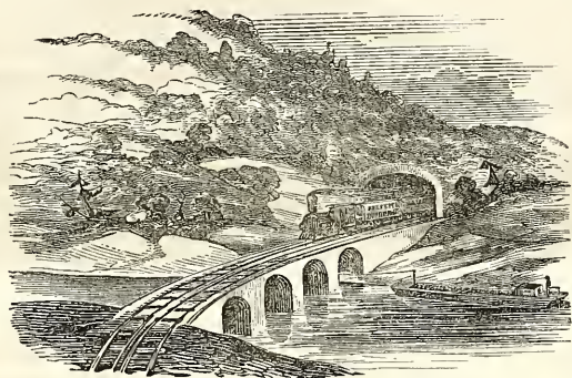
TUNNEL AND BRIDGE ABOVE PHENIXVILLE.
